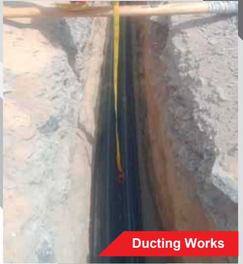
Ducts Laying at Mountains
