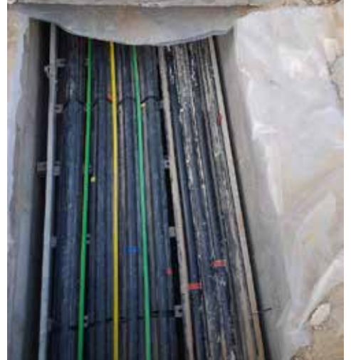
Cable laying through trenches
