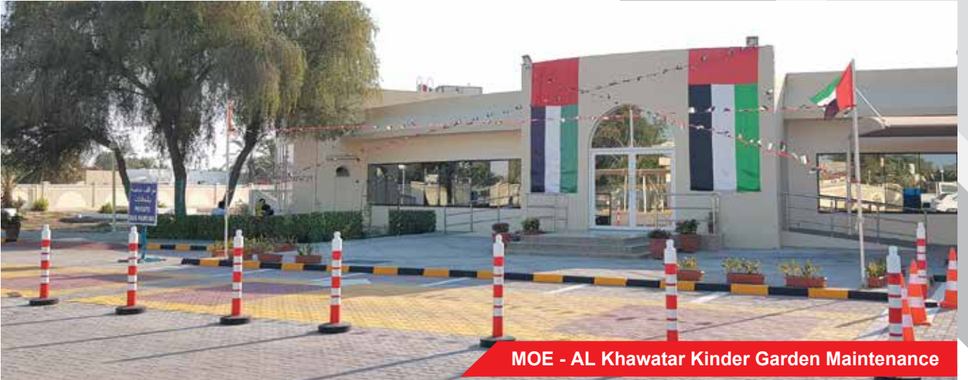
MOE - AL Khawatar Kinder Garden Maintenance
