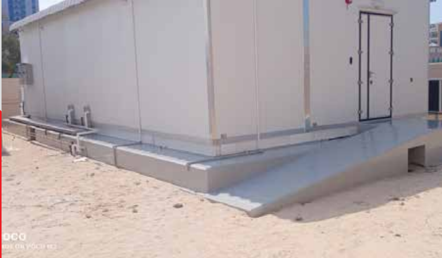
Mega shelter foundation at Etisalat Exchanges
